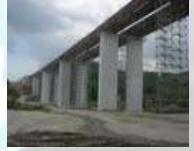
Subic Clark Tarlac Expressway
