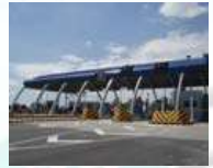
North Luzon Expressway
