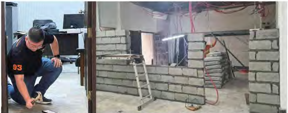
Left: M.Ed. WB Raymond Wong, performs a simple Feng Shui ritual to symbolically commence construction. Right: The TCT Office at the height of the renovation works.
