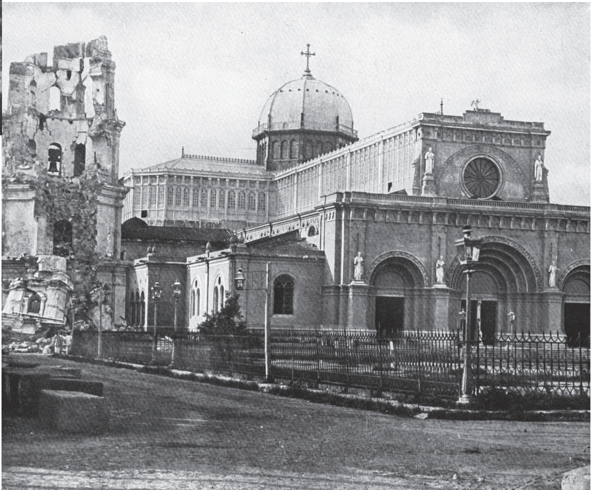
Manila Cathedral after the June 3, 1883 earthquake. The cathedral's stand-alone bell tower was toppled down by the powerful tremors just as parts of the city and the suburbs had been leveled to the ground.
