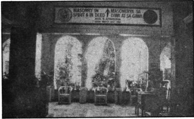
Present lobby at the old Plaridel Temple building.
