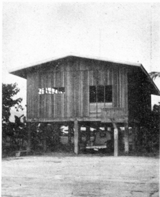
Temple of Agno Lodge No. 75 in Ta- yug, Pangasinan under construction.
