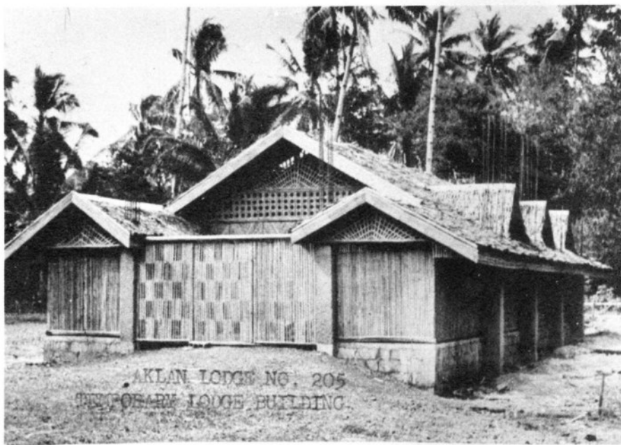
Temporary Lodge Building of Aklan Lodge No. 205 in Kalibo, Aklan constructed on the foundation of the proposed Lodge Temple.
