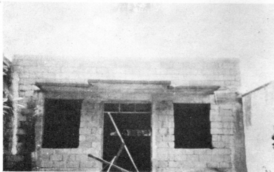
Temple of Plaridel Lodge No. 74 in Calauag, Quezon under Construction
