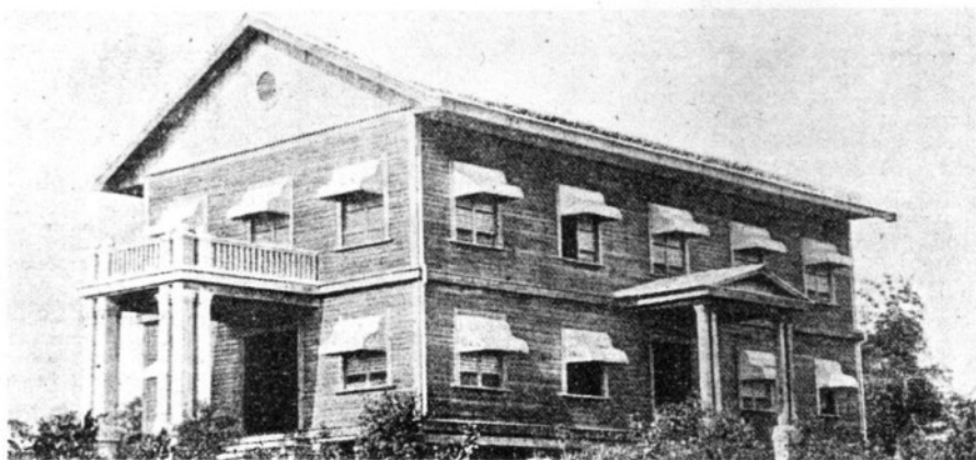
OLD HOME OF MALINAW LODGE NO. 25 San Pablo, Laguna
