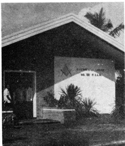
Facade of new Makawiwili Lodge Hall.
