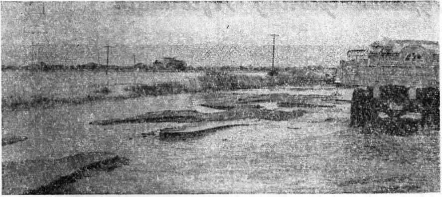
Road conditions in Central Luzon after the flood.
